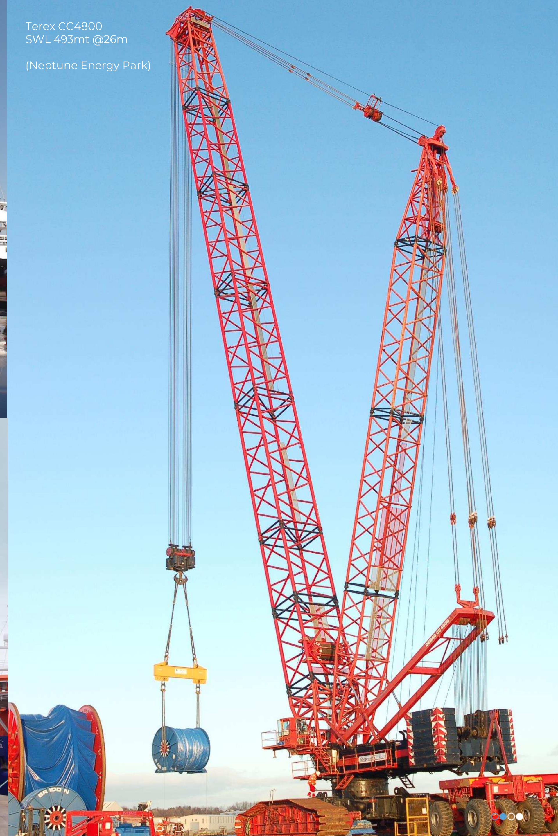
325t Hammerhead Crane SWL 325t @24.5m (Offshore Tech Park)
